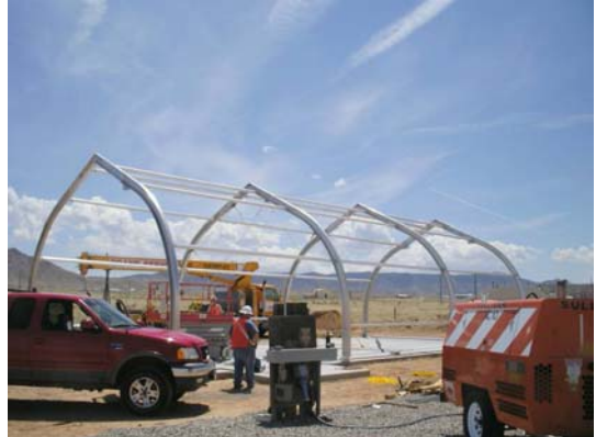
Figure 20 and Figure 21 – Sprung Structure Aluminum Inner Frame Installation and Completion
