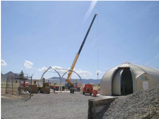
Figure 20 and Figure 21 – Sprung Structure Aluminum Inner Frame Installation and Completion
