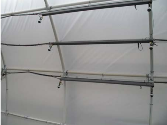
Figure 28 – Three Modular Spray Booms
