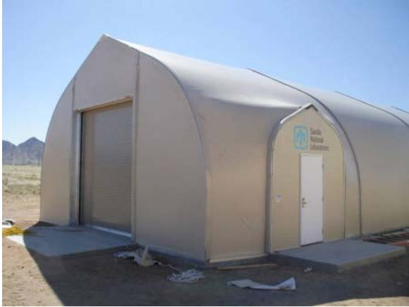
Figure 23 – Sprung Structure Installation Complete
