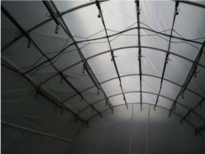
Figure 25 – Photo of Spray Nozzle Assembly Installed Within Tented Operational Geometry
