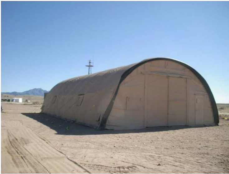
Figure 18 – Front View of CAMSS30 at Sandia Location
