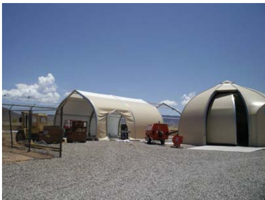
Figure 22 – Sprung Structure Membrane Liner Installation
